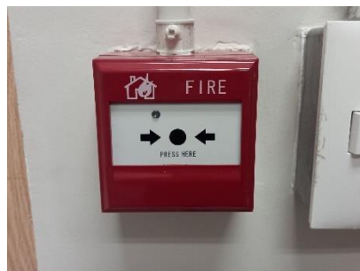
Fire Alarm Manual Station
