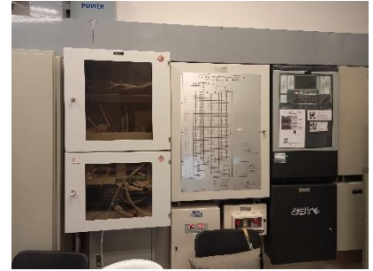
Graphic Annunciator Fire Alarm System
